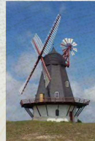
Smock Mills who had strong base and wooden body which also featured rotating roof.
